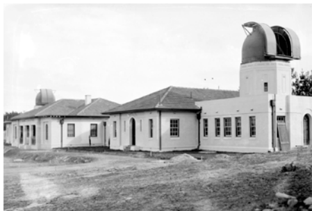
Solar Tower, Observatory offices and buildings, six-inch Farnham Telescope, Mount Stromlo Observatory. Circa Jan 1921–Dec 1935.
